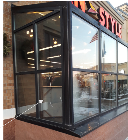
Broken Glass due to settling issues
