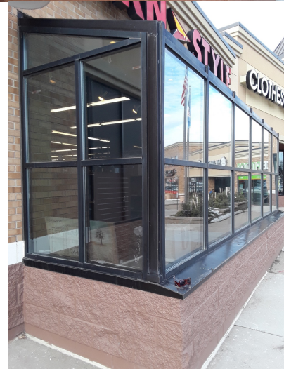
Brin Glass Service Glaziers made the repairs necessary
